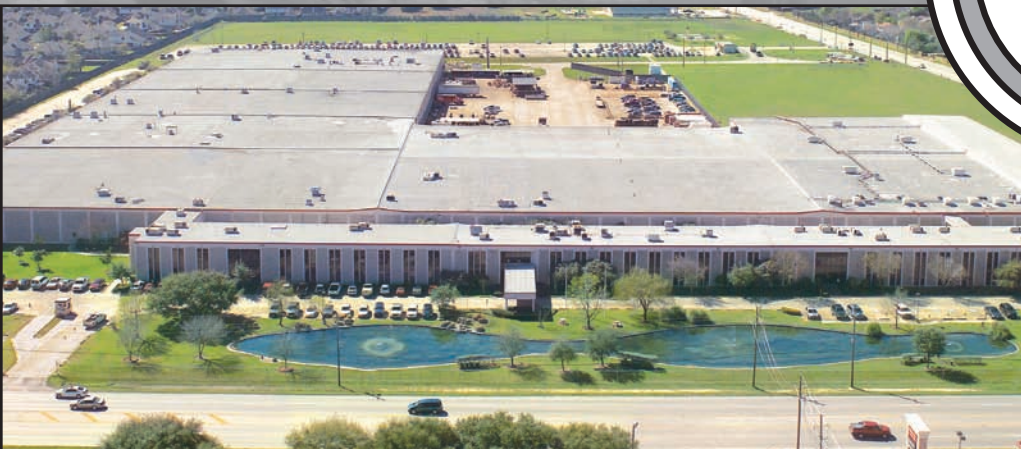
North American Headquarters & Manufacturing Facility (Houston, TX)
